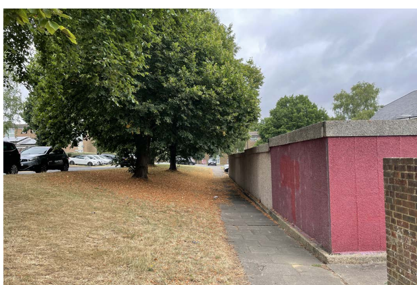
Image 3 :View of the sloped landscape
