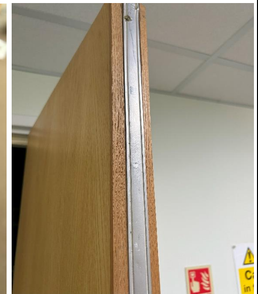
No intumescent strips or cold smoke seals. Door opens onto a means of escape.
