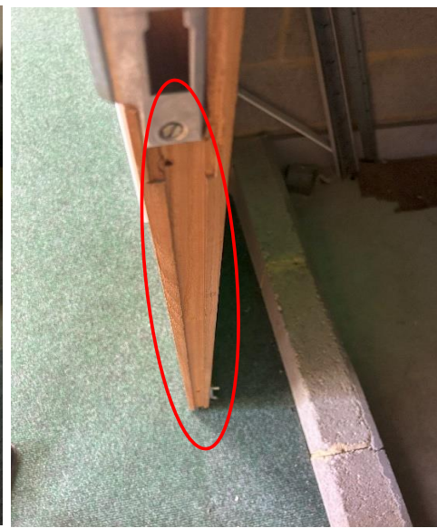
Missing/damaged intumescent strips and/or cold smoke seals. Doors open onto a means of escape.
