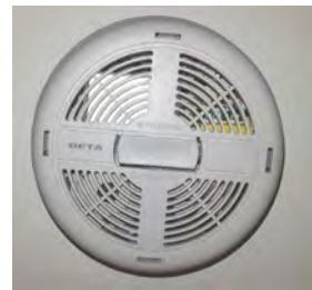
Smoke alarms are mounted on the ceiling within the entrance hall on the ground floor and on the first floor landing. These are linked so if one is triggered both will sound.
