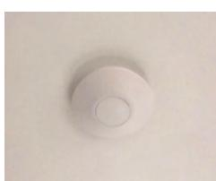
The kitchen and bathroom are fitted with Mechanical extract ventilation units. The system runs continuously providing a comfortable level of 'background' ventilation which can be manually boosted when cooking or bathing/showering to help clear moisture-laden air. To prevent excessive condensation, and possible mould growth, the system should NEVER be switched off unless servicing the fan units.
