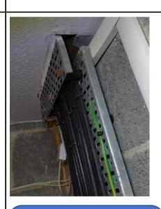
Fire stopping is required to prevent the spread of smoke, gases and fire from one compartment to another.
