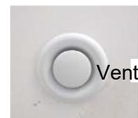
A boost button (Fan boost) can be used when using the bathroom or cooking. This may be a standard switch or a square panel which uses 3 for boost and 1 for off.
