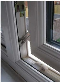
Most windows above ground floor have over-ridable restrictors. There are width restrictors fitted to all upstairs windows. Open these by partially opening the window and gently pushing the catch down.
