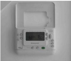
The heating and hot water systems are controlled by a programmer that allows you to switch your system on and off at times that suit you. Your home has two programmable zones, so you can set the heating to come on and off at different times for upstairs and downstairs.
